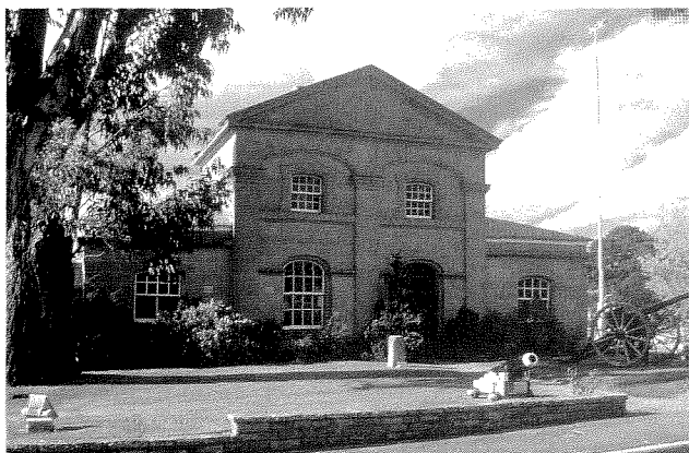
Figure 4. Anglesea Barracks Military Prison, front or southern elevation—originally Provost's Quarters. (Photograph taken by, and courtesy of, Ivar Nelsen, 1987.)
