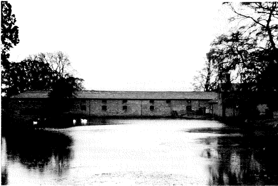
Fig. 9: The dominant method of water supply for mills in Britain was direct from large ponds, as seen here at Shugborough Mill, near Stafford (photo. Pearson 1992).
