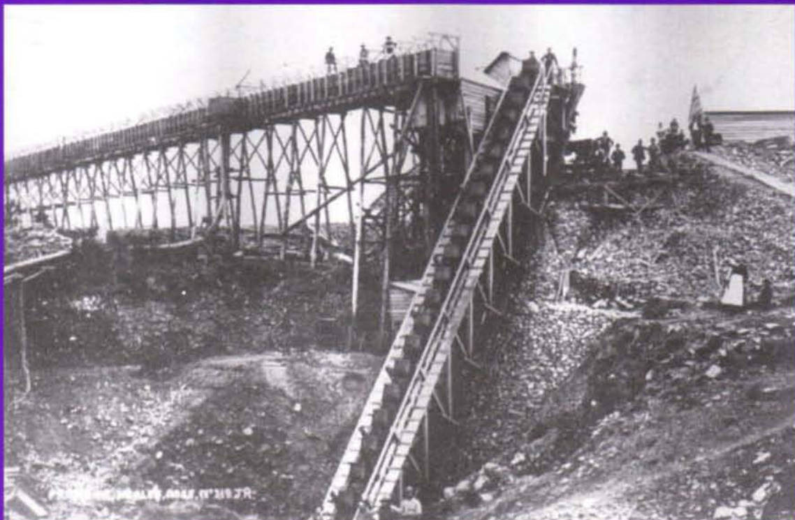
A bucket elevator on the Ross goldfield, West Coast, South Island, New Zealand
