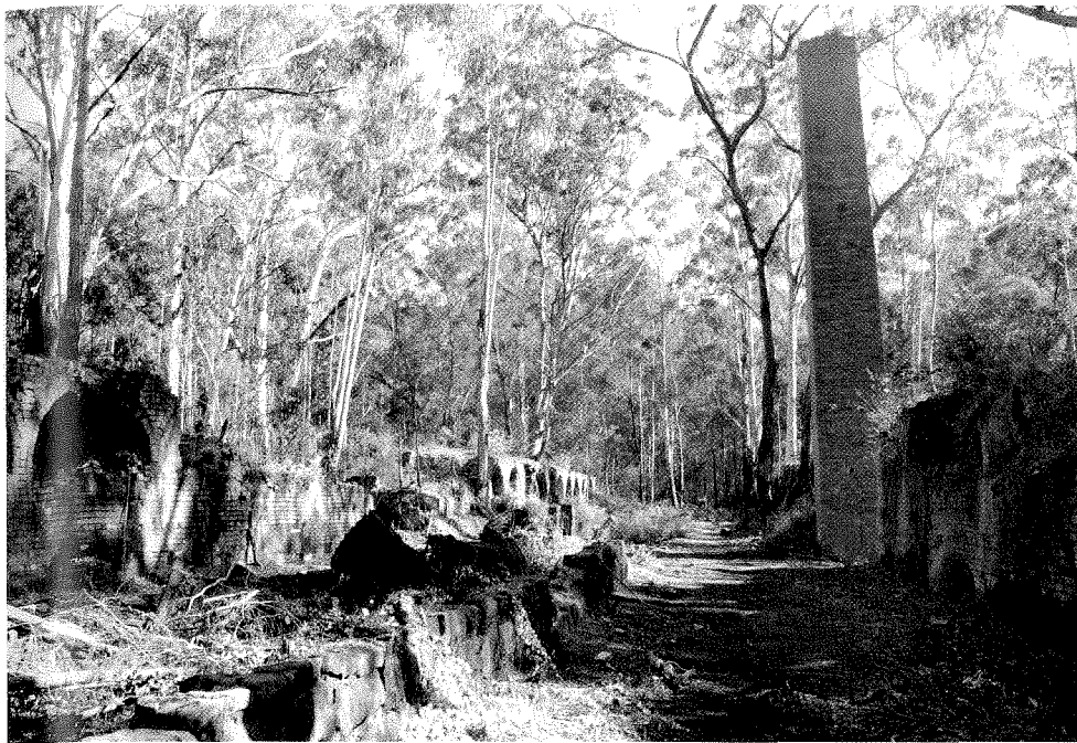
Fig. 4: The four benches of retorts with the surviving chimney-stack, from south-east. The volatilised oil from the retorts was condensed in the central area and piped down to the refinery. (R. Ian Jack, 1995).
