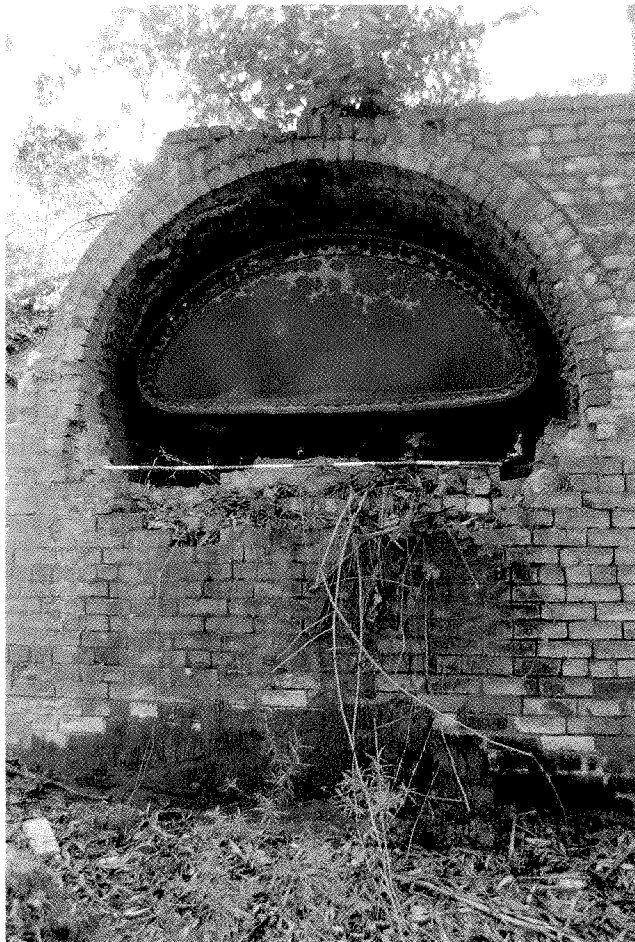
Fig. 5: A retort in situ, showing the sealed end. The arch was bricked in during use but allowed the pipe carrying the volatilised oil to pass through. Scale 10 x 20 cm. (R. Ian Jack 1995).
