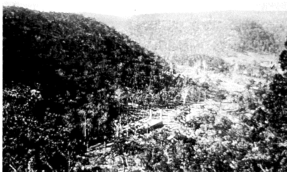
Fig. 3: The first two benches of retorts at Joadja photographed in 1879, showing the physical context in Russell's Gully. The oil-shale mines are high up on the surrounding cliffs, the refinery site to the middle right.
