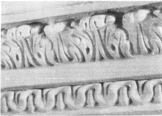
Fig. 7: Hall cornice, c.1860, Margareta Cottage, Glebe.
