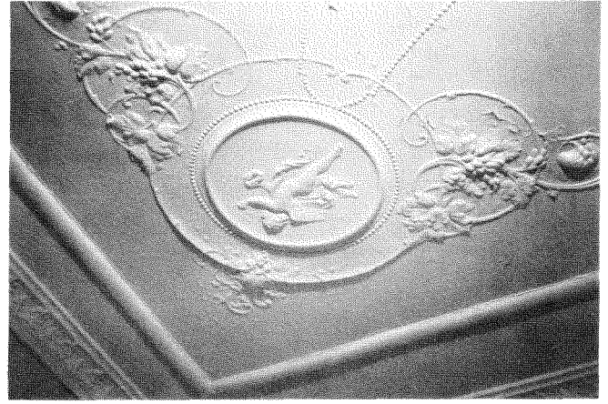
Fig. 16: A scantily clad putto holding a victor's wreath frolics among vine tendrils on a 1930s fibrous plaster ceiling panel.
