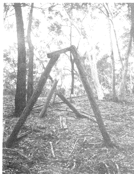
Fig. 11: Wattle Flat: trestles leading into (from) the dam.
