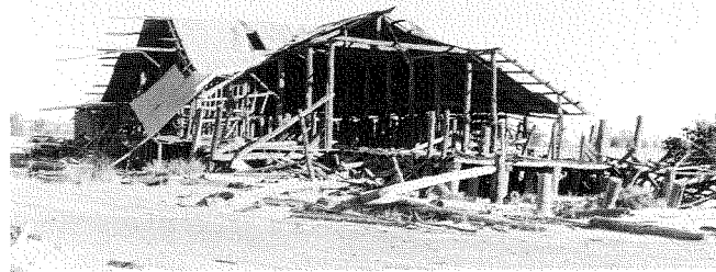
Fig. 2: Wooyeo woolshed. This T-shaped structure was built in 1873 with 52 stands to shear 100,000 sheep each year and includes such details as sliding gates and trapdoors to encourage a smooth work flow as well as ample sheep shelter and wool storage space. It now serves multiple storage purposes on a small farm as it gradually melts into the surrounding wheat paddocks.
