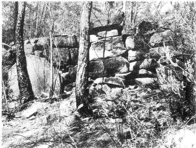
Fig. 5: Type 1b stonework in the Sampson's Pass area, 35.2km north of Wisemans Ferry. The stones are approximately 30×30–90×30cm. (Photograph by G. Karskens.)
