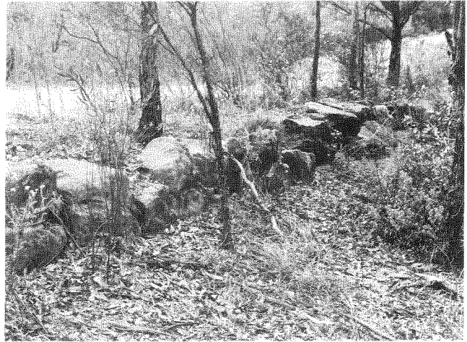
Fig. 4: Type 1a stonework on a low embankment, at the summit of Devine's Hill, 2.95km north of Wisemans Ferry. The stone-sizes vary around 30×50×30cm. (Photograph by G. Karskens.)
