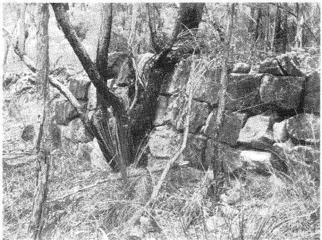
Fig. 6: Type 2a stonework, showing rough shaping and intermittent coursing, 7.9km north of Wisemans Ferry. The stones are approximately 15×30×15cm. (Photograph by G. Karskens.)
