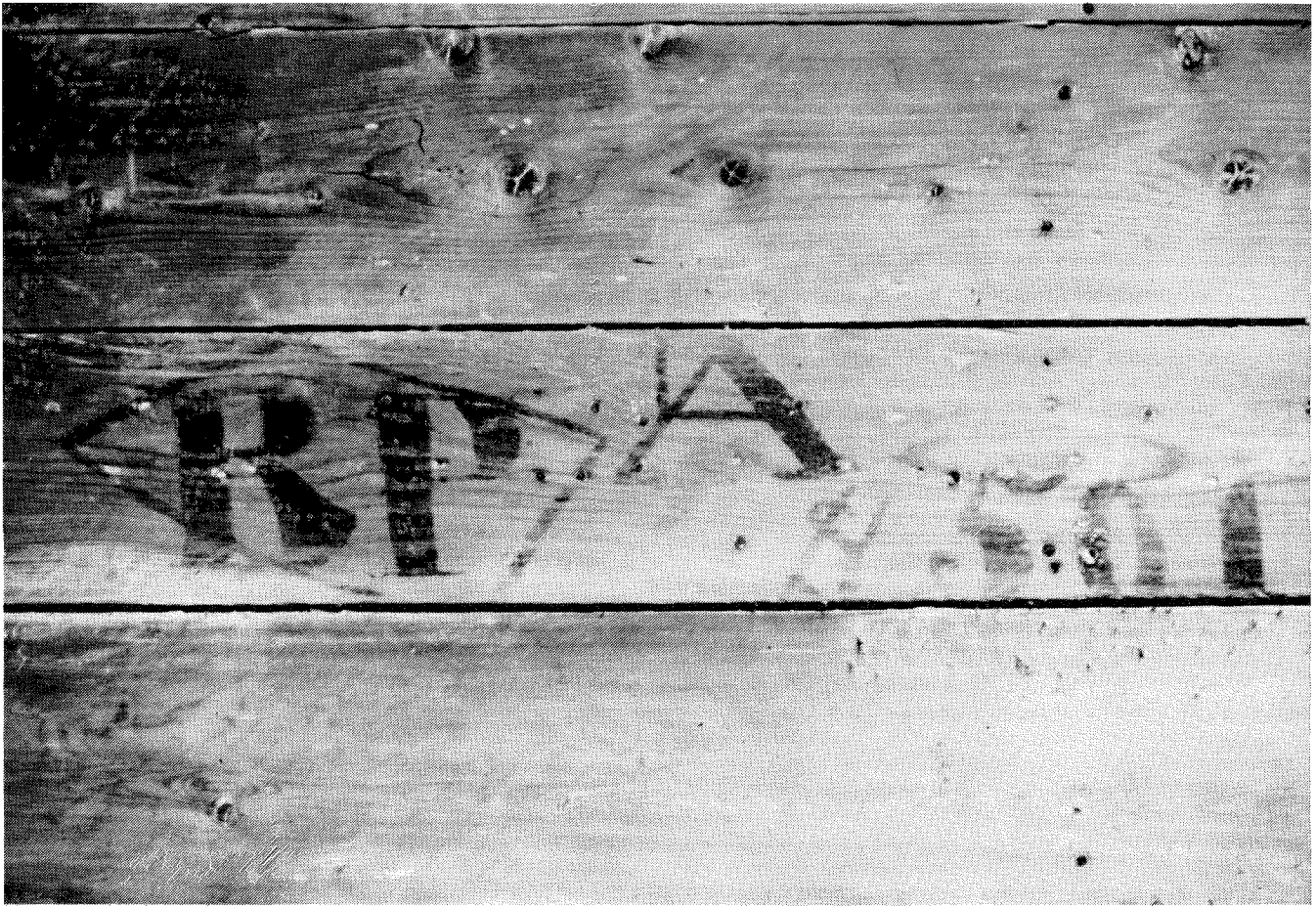
Fig. 2: 399 Coventry Street, South Melbourne, c.1853: detail of the lining boards, probably used previously to crate the building materials. In the lading mark 'R.P.' stands for Robert Patterson, the consignee. Photo: author.
