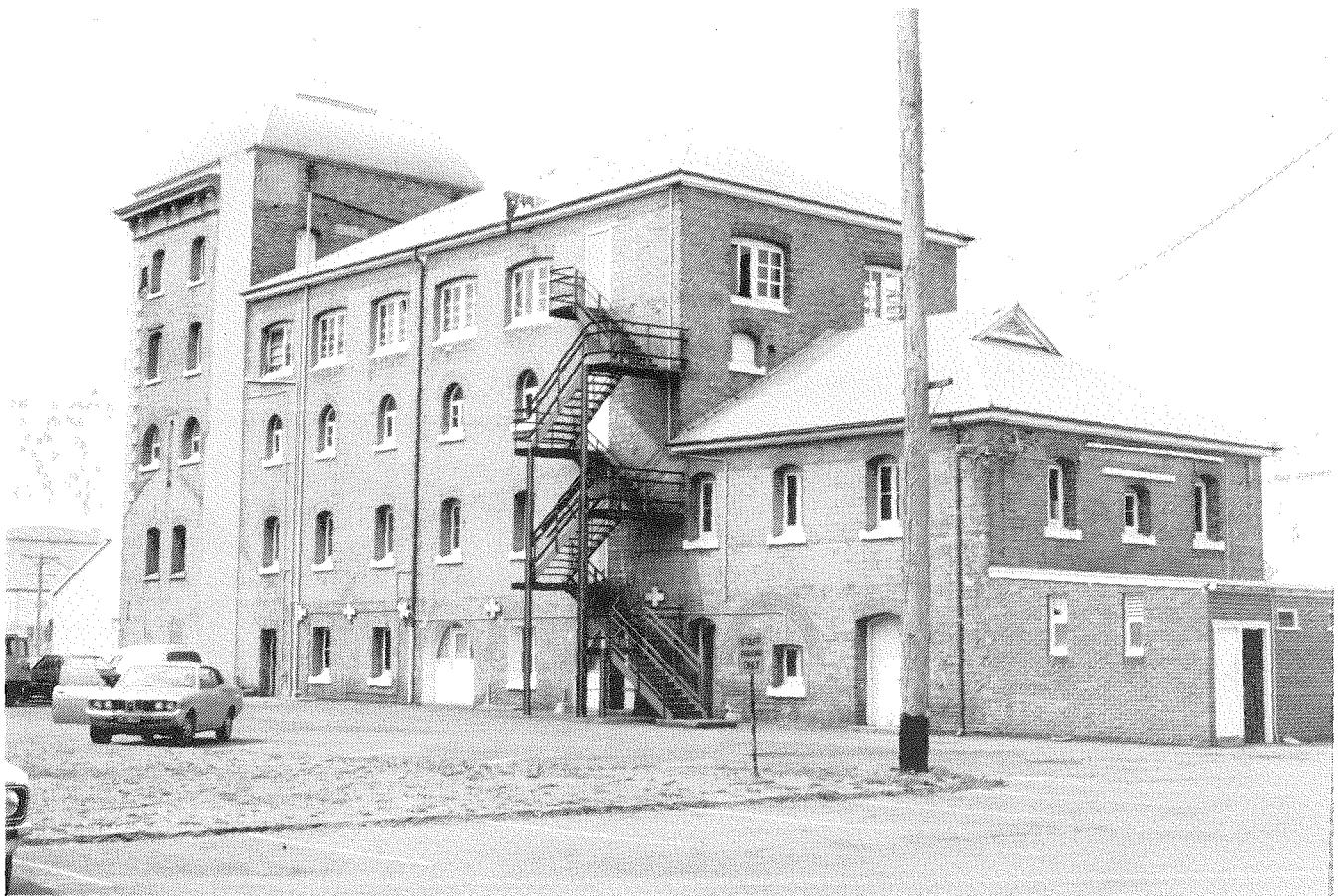
Fig. 7: The west side of the Great Northern Brewery, 1979.
